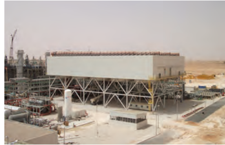
Hassi R'Mell, Algeria — ACC for 150 MW Combined Cycle Power Plant – Solar Power Plant.
