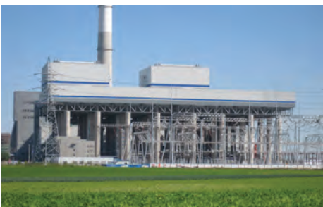
Baicheng, China — ACC for 2x660 MW Coal Fired Power Plant.
