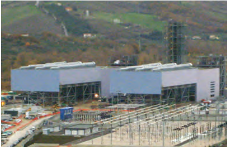
Gissi, Italy — ACC for 2x400 MW Combined Cycle Power Plant.
