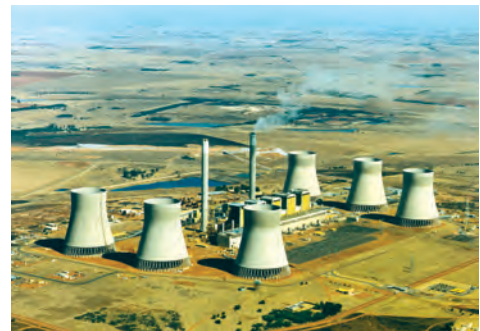
The world's largest Natural Draft Dry Cooling System, 6 x 690 MW Kendal Power Station, South Africa
