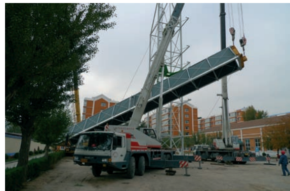
A 25m high MegaDelta being lifted
