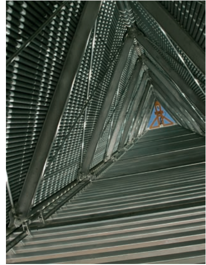
Inside view of MegaDelta during lift
