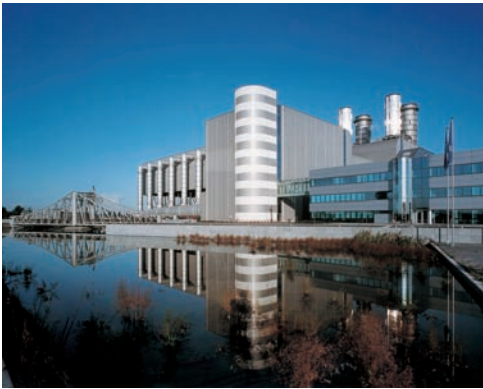
460 MW Combined Cycle Power Plant Bruges, Belgium
