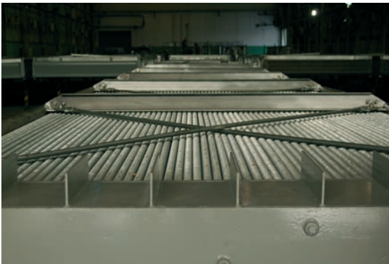
Finned tubes being welded to the tube sheet
