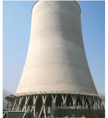
2 x 660 MW Coal Fired Power Plant with FGD Qinling, China – 2011
