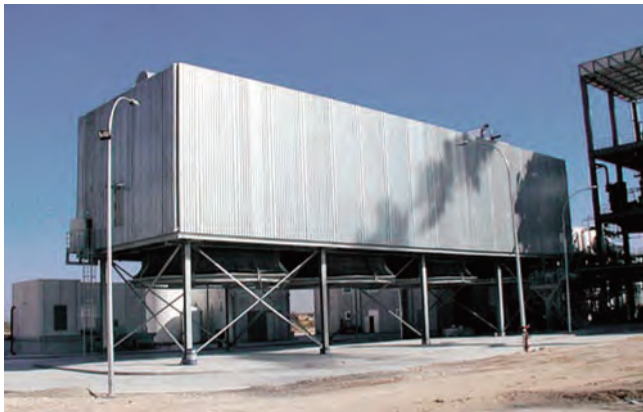
A-Frame ACC installed in a 15 MW Power Plant fueled with Dry-Waste Biomass from the Olive Oil Industry in Spain
