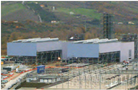
Gissi, Italy — ACC for 2x400 MW Combined Cycle Power Plant.
