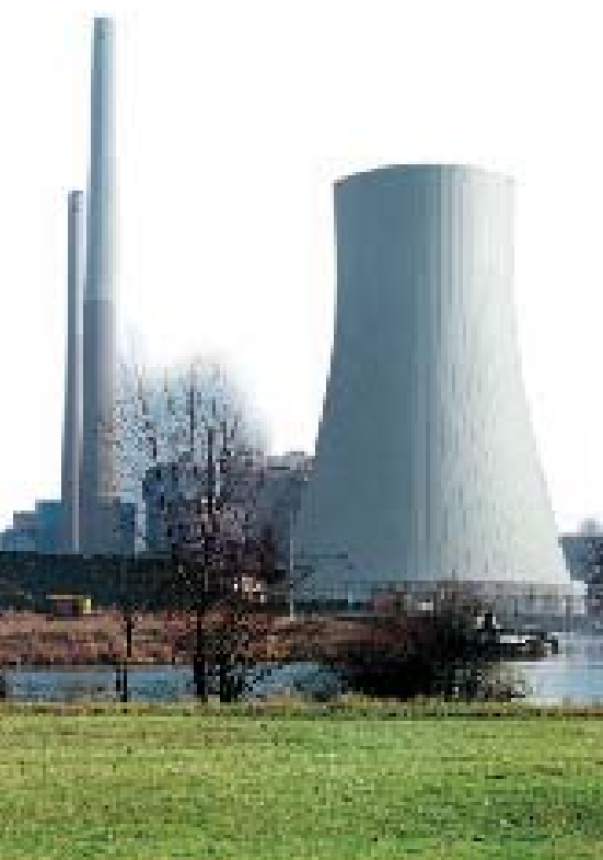
Natural draught cooling tower at a large power station: sound attenuators at the air inlet reduce sound emissions
