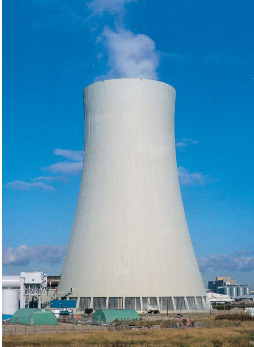
Cooling tower simultaneously used to discharge treated flue gases from the 550 MW power generating unit of a coal-fired power station
