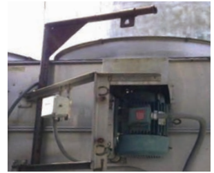
Other manufacturer's booms are fixed to only reach the motor.
