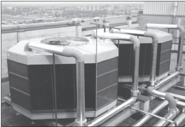
A modern cooling tower developed through use of CAD/CAE features construction materials of fiberglass, stainless steel and PVC.
