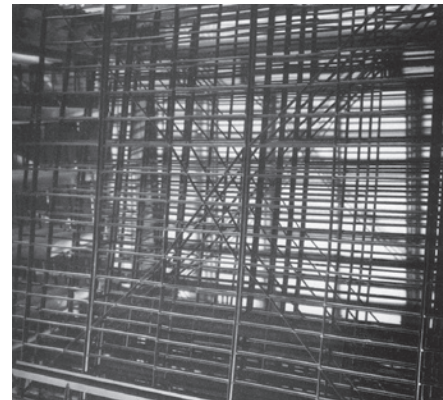
Ladder crossflow polypropylene splash-fill
