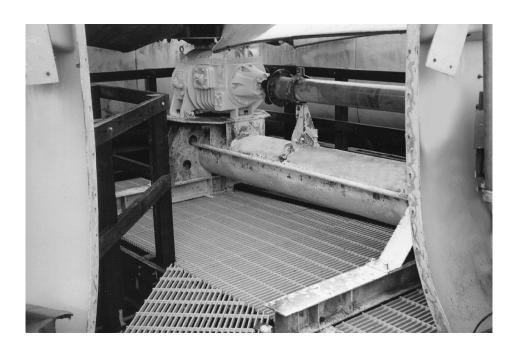
For permanent equipment access walkways or temporary work platforms, fiberglass grating assures premium performance. It's corrosion-resistant, slip-resistant, strong, ultraviolet-resistant, lightweight, and fire-retardant.
