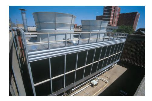
The Marley Sigma F series crossflow cooling tower utilizes advanced composites and stainless steel for excellent durability and corrosion resistance in a truly cost-effective design.
