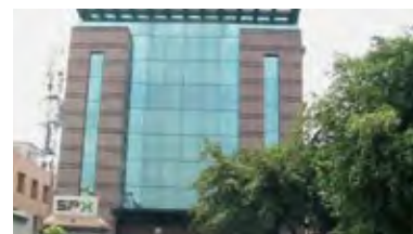
Service Solutions validation center in New Delhi
