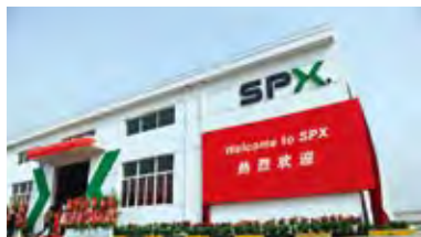
SPX (Shanghai) Flow Technology Co., Ltd.
