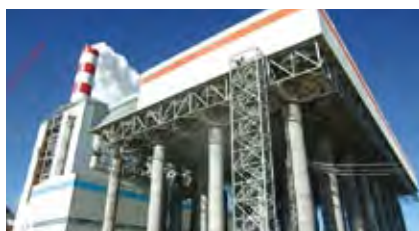
Air Cooled Condenser
