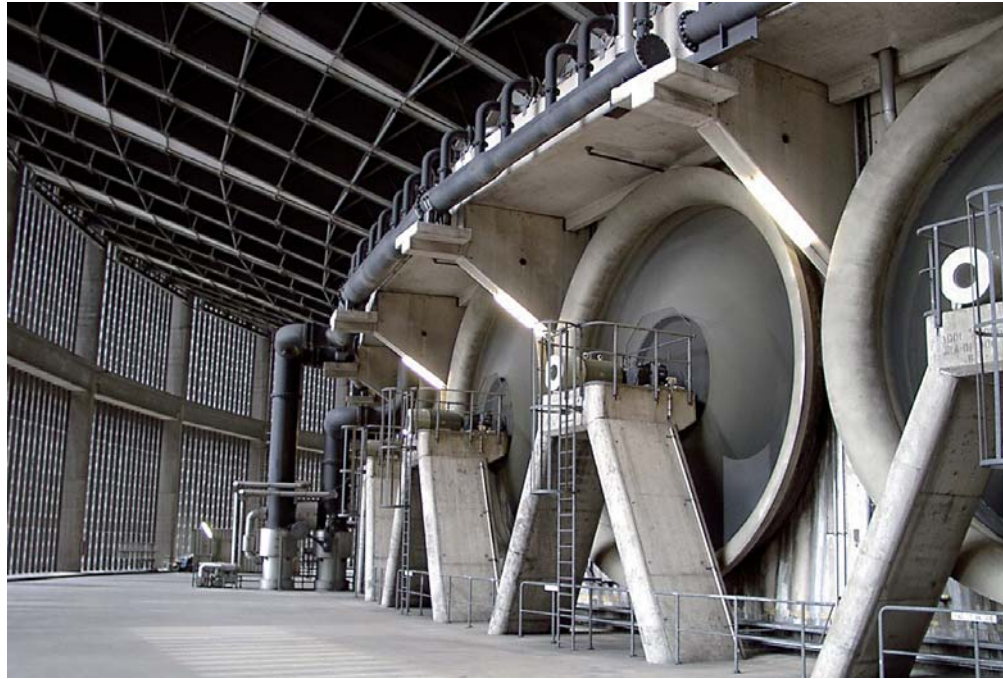
Low-noise fans developed at SPX Cooling Technologies
