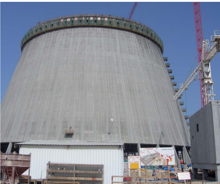
Circular cooling tower under construction
