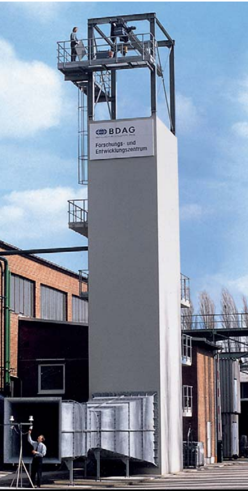
Test cooling tower at SPX Cooling Technologies' research and development centre
