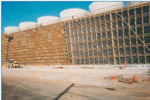
Replacing louvers
