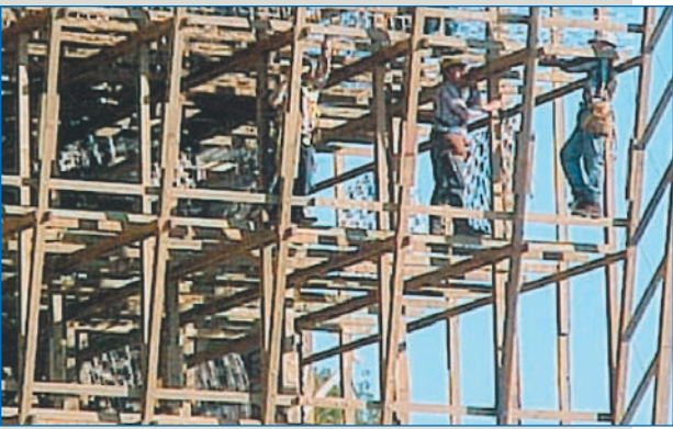
Structural upgrade of a wood tower
