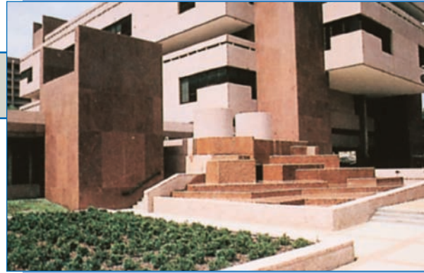
MS concrete tower designs enhance the surrounding architecture
