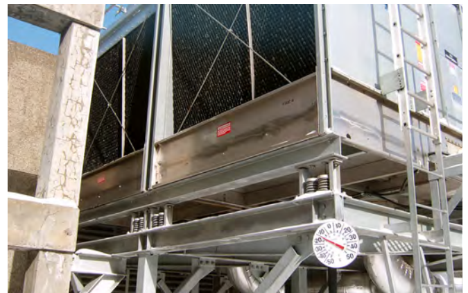
Cooling tower operation at -15^{\circ}\text{C} — slight visible ice
