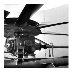
Gear reducers shall meet or exceed the requirements of CTI STD-111 and AGMA Std. 420.04, and service factor at applied horsepower shall not be less than 2.0. They shall be run at the vendor's factory under load to verify acceptable service, and to coat the interior surfaces with a rust-proofing oil prior to shipment.
