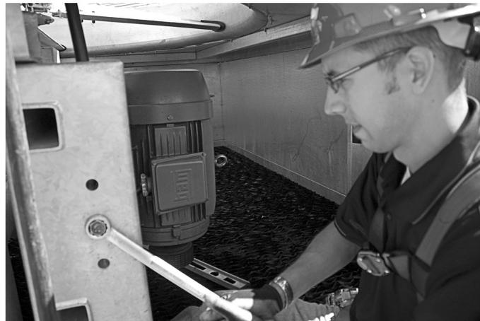
New belts (operating less than 8 hours) should be tensioned to the maximum value. Tension after this period should use no less than the minimum value. If the belt span was measured in inches, then use the pounds of force values. If the belt span was measured in centimeters, then use the kilograms of force values. If specific tensioning instructions are provided with your tensioning tool, those instructions should be used instead.
