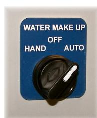
The water makeup selector switch is located on the right-hand side of the enclosure.
