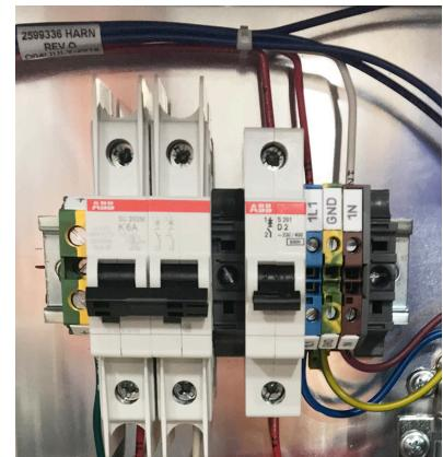
2. Power ON the control panel circuits by switching both circuit breakers to the up position.
