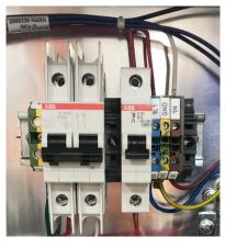
2. Power ON the control panel circuits by switching both circuit breakers to the up position.
