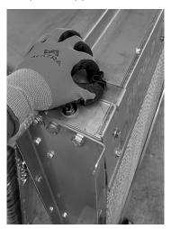
2 Rotate the retainer clips 90° to free the upper basin. Next, rotate the basin upward so pad can be removed.
