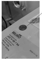
Manual Override Button Must be Flush with Top of Cover
