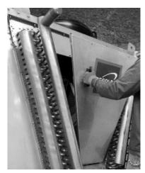
Remove all of the shipping wires between the interior X-bracing. Cut and discard. Re-install access door when complete.
