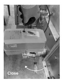
4 Verify that the manual override button pops up flush with the top of the cover after work is complete. It may be necessary to rotate the button counterclockwise using the screwdriver to free the button from the locked position.
