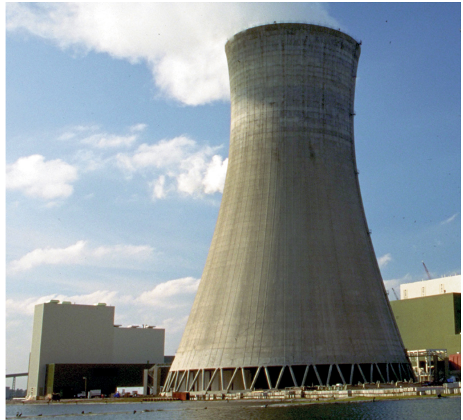
Natural-draft cooling tower – field-erected (FEP) counterflow cooling tower
