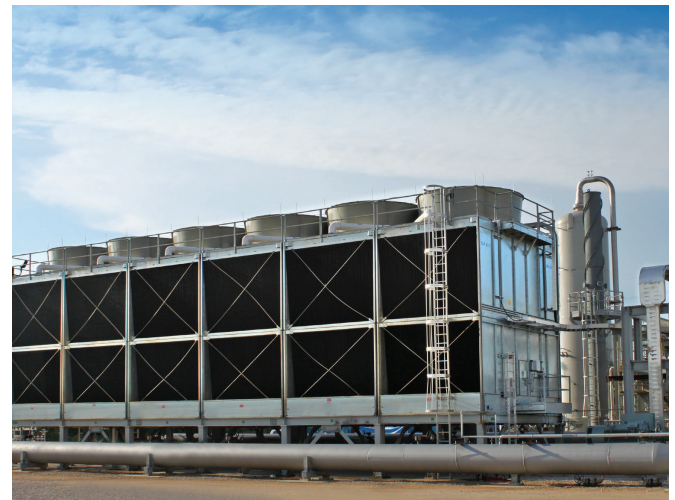
Factory-assembled (FAP) cooling tower – induced-draft crossflow cooling tower
