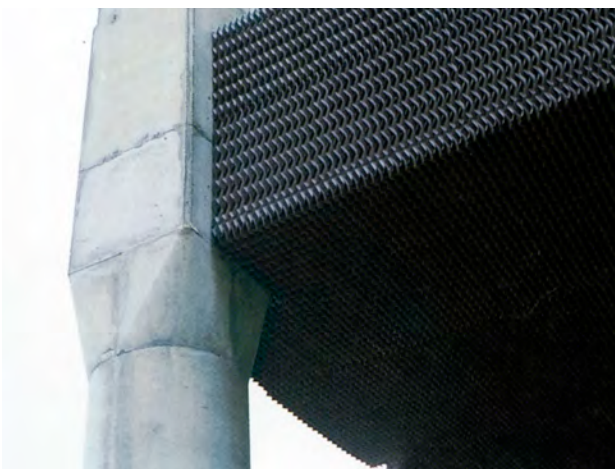
Unobstructed Marley counterflow fill installation
