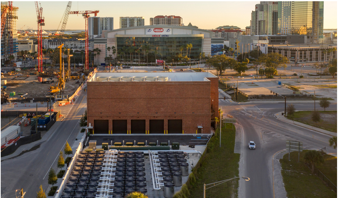
The bank of six Marley NC Cooling Towers are housed in a brick building facade. The fan cylinders are barely visible from this elevated view.
