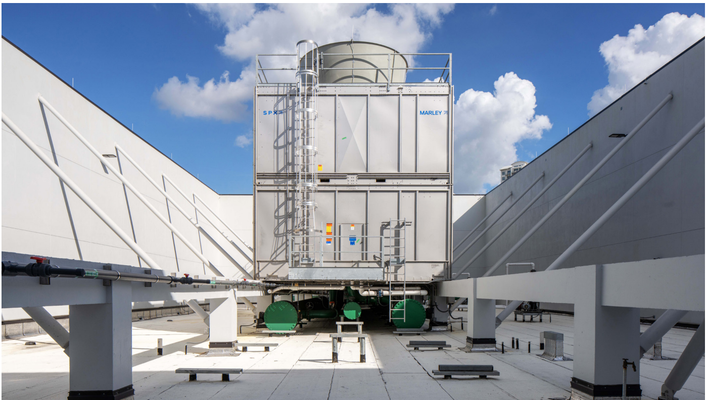
Marley NC Cooling Towers provide over 8000 tons of cooling capacity.
