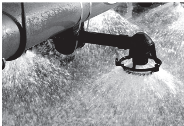
Figure 57 — Counterflow distribution system in operation
