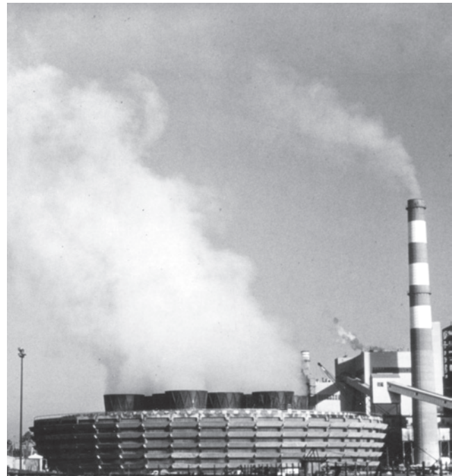
Figure 32 — Round mechanical draft tower operating in a significant wind. Compare plume rise to flat trajectory of smoke leaving stack.
