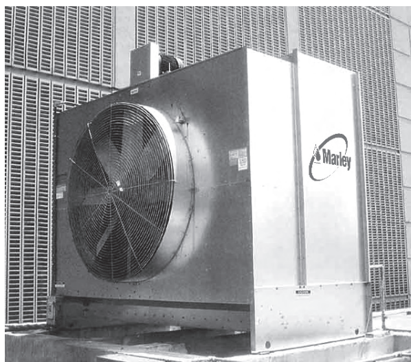
Figure 11 — Small factory-assembled tower.
