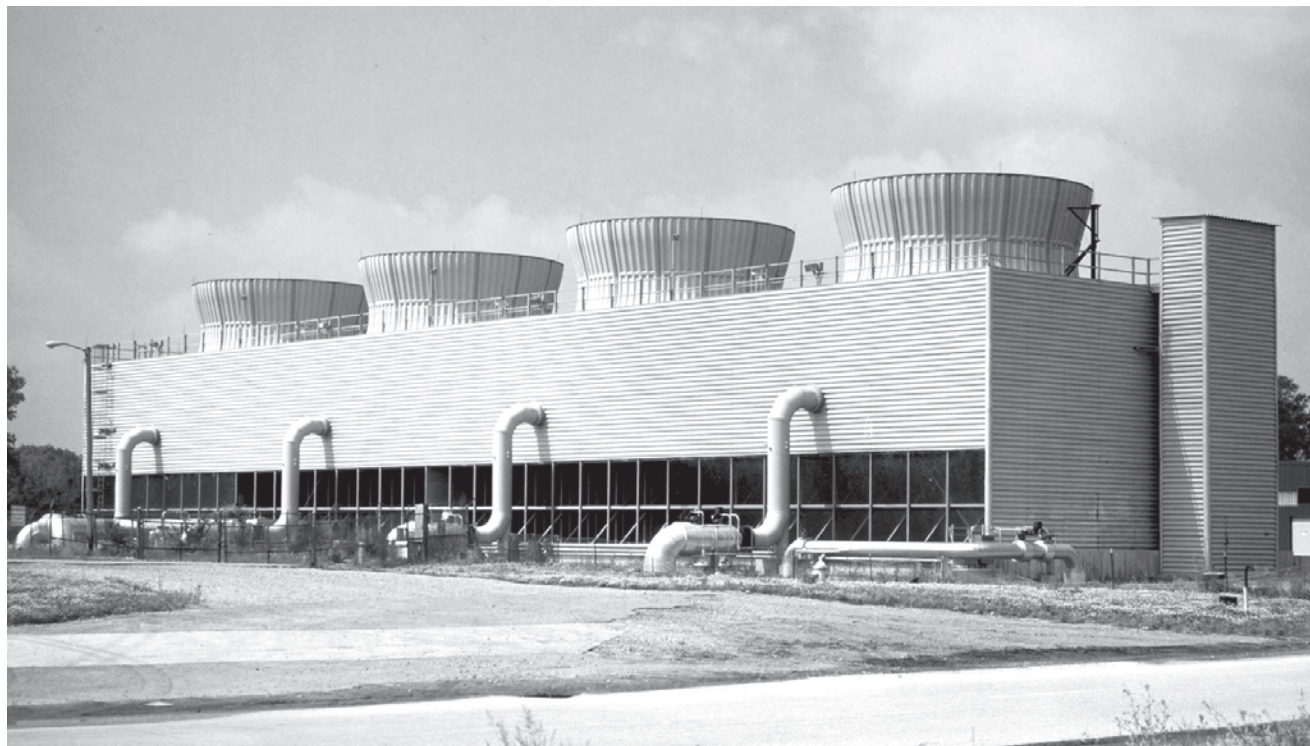
Figure 58 — Four-cell tower with individual side risers.
