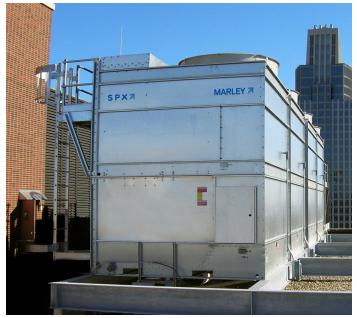
**MARLEY AV CROSSFLOW COOLING TOWER** Singleflow, induced-draft design offers pump and fan energy savings in a small footprint. Factory assembly and G-235 galvanized steel construction are standard. Tower capacity from 125 to 772 tons per cell. CTI Certified.
