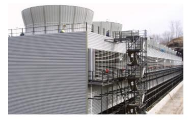
**MARLEY PPWD HYBRID PLUME ABATEMENT COOLING TOWER** The parallel-path/wet-dry hybrid cooling tower offers efficient cold water temperatures with reduced visible plume and enhanced water conservation.
