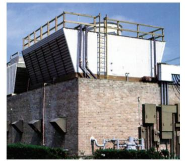
**MARLEY SERIES 10 - SERIES 15 CROSSFLOW COOLING TOWER** Splash-fill design for use at high temperature or where poor water quality prevents the use of film fill. Treated wood structure. Tower cells available from 135 to 6,720 gpm.
