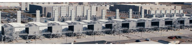
Energy savings HVAC evaporative cooling systems can reduce energy consumption by one-half to one-third, compared to air-cooled equipment. (Results are climate and water resource dependent.)
