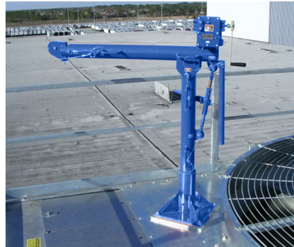
Boom reaches over NC fan deck railing and fan
