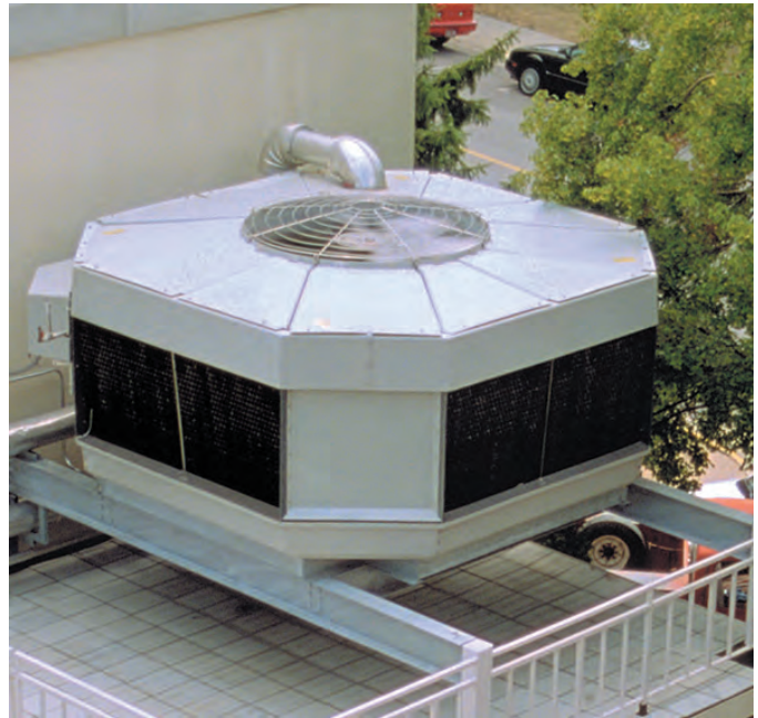
Stainless steel, FRP and PVC make this cooling tower virtually corrosion proof
