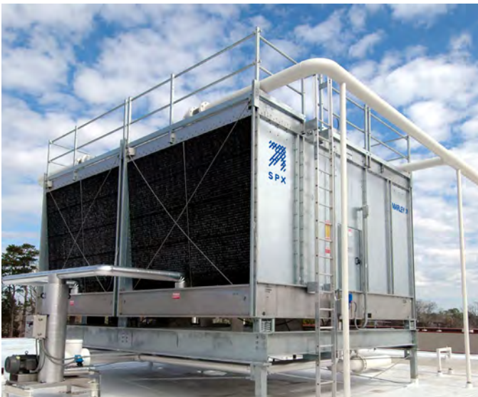
Steel structure and casing in a crossflow design
