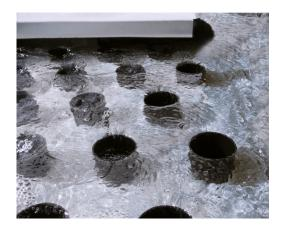
Marley-engineered Low-Flow Nozzle Cups can effectively divide the hot water distribution basin into outboard and inboard sections, allowing the cooling tower to manage variations in flow automatically while maintaining adequate head over active nozzles. Most importantly, uniform air-side pressure drop is maintained across the fill with the MarleyGard Low-Flow Nozzle Cups. Additional benefits include:
