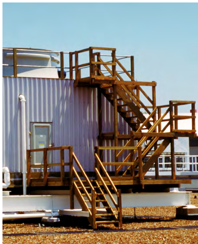
Wood Stairway with Access Platform
