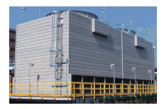
Marley DuraLast™ pultruded fiberglass architectural casing is an attractive, ideal material for the wet, corrosive cooling tower environment. It's strong and lightweight. Plus, it will not corrode from chemical exposure or moisture, and it resists deterioration from sunlight.
