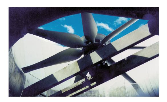
The HP7000 fan is designed for industrial cooling tower applications, offering distinct advantages over other fan designs. The Marley FlareTip™ blade enhancement provides increased performance overcoming tip clearance losses—aiding the movement of air next to the fan cylinder.
