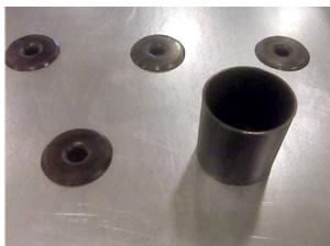
Simple modifications to Marley crossflow cooling towers permit variance in the flow rate over a wide range by varying the number of nozzles that are active as a function of the flow rate.
