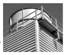
■ This "side inlet" method of piping the cooling tower requires you to provide a header at the base of the tower, along with separate risers for each cell. Using this method, you may conveniently valve off cells on an individual basis.
