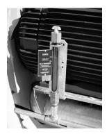
Fans of the size used on large cooling towers are applied at speeds and horsepowers that generate considerable torque—and structural tubular steel resists this torque very effectively. The Marley torque-tube assures that all of the mechanical equipment remains aligned, and that the rotating fan is properly positioned within the fan cylinder. Hot-dipping after fabrication assures that all steel surfaces will be heavily coated with zinc for long-term protection against corrosion.
