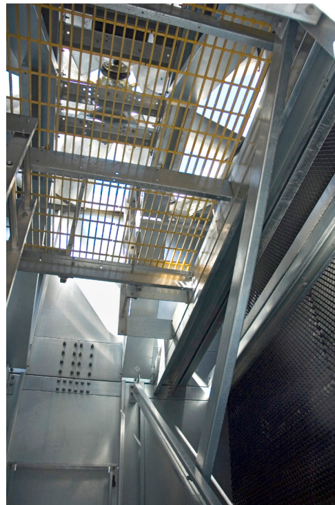
Mechanical Equipment Access Platform
