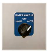
is filled, the switch is placed in the AUTO position to allow the adjusted probe assembly to monitor and sustain the proper operating level. Placing the switch in the OFF position completely interrupts any monitoring or fill action normally provided by the LLC control panel. Normal tower operation depends upon the HAND-OFF-AUTO switch being positioned in the AUTO mode at all times.
