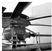
Many of the large fans used on cooling towers operate at tip speeds approaching 13,000 ft/min. When the blade tips encounter the occasional solid droplet of water that escapes the eliminators, erosion of the leading edge can occur on fans whose designs do not address this problem. This has, over time, contributed to some fan failures in the past.
