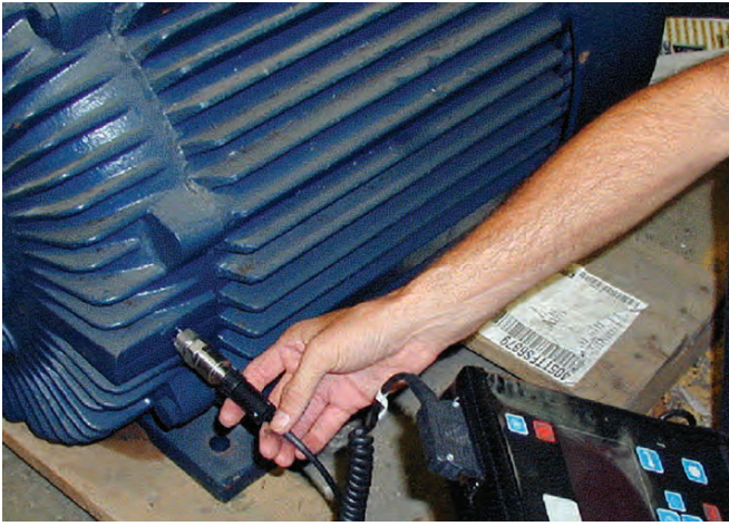
Use a handheld vibration monitor to check mechanical operation
