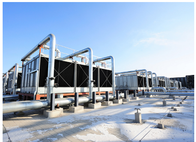
Evaporative cooling towers are an integral part of many data center cooling systems.
