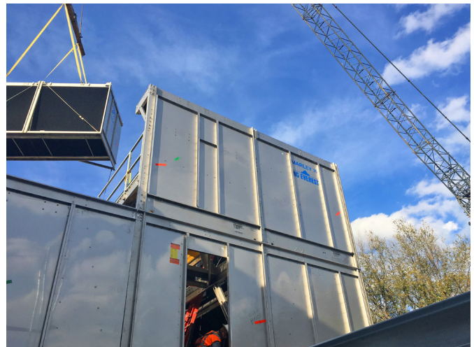
The next generation of factory-assembled cooling towers can be delivered up to 60 percent faster than field-erected towers and installed 80 percent faster.
