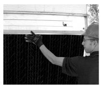
Collection basin floor has uneven surfaces and has the potential to be slippery. Care should be taken if entering the basin. Louver edges can be very sharp and could cut skin if proper protection is not used. Always wear gloves and sleeves when handling
