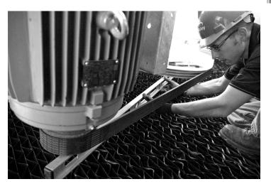
The number of grooves on the motor and fan sheaves may not match each other, or the number of grooves on the belt. Always install the belts on the highest grooves on the fan sheave. Doing so will reduce the force on the fan shaft bearings, thus increasing their life.
