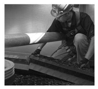
To remove the eliminator, stand inside the access panel and lift with two hands on an eliminator section, this will indicate where one section stops and another starts. Lift the eliminators at that intersection, removing two packs at one time (see image). Once the first two packs are removed, the remaining packs should
