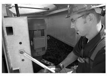
New belts (operating less than 8 hours) should be tensioned to the maximum value. Tension after this period should use no less than the minimum value. If the belt span was measured in inches, then use the pounds of force values, see the following table. If the belt span was measured in centimeters, then use the kilograms of force values.
