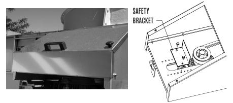
On 8.5' wide models, the fan motor and belt adjustment mechanism is located outside the fluid cooler. Remove the motor protection hood by loosening the two thumbscrews on top and hinge the hood up and out of the way. Also, remove the motor sheave safety bracket and set aside. See the following images. On 10' and 12' wide models, the motor is located inside the fluid cooler plenum. Open the access door (see Access Door Operation) and hinge out of the way.
