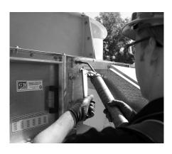
**Semi-Annually** If equipped, check the belt tension and condition. Adjust tension as necessary.
