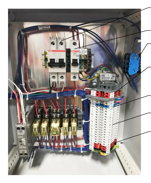
Route incoming power cable from the bottom of the enclosure up into the top (line) side of the main circuit breaker.
