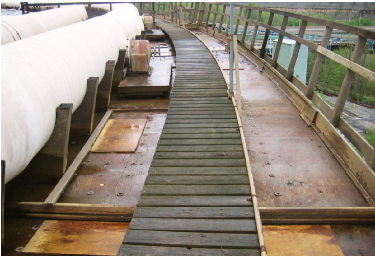
Wood Crossflow Cooling Tower Prior to Reconstruction
