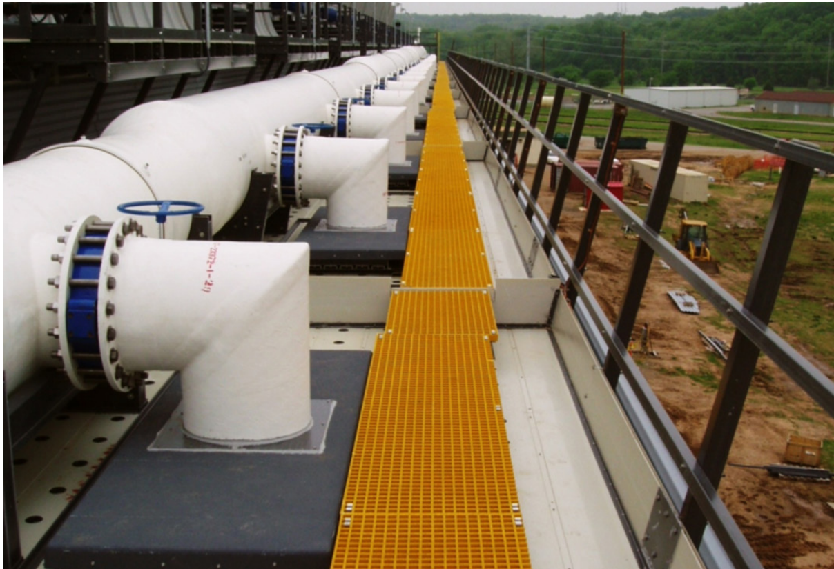
Post-Reconstruction Showing FRP Structural Enhancements
