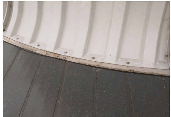
Reflex RTM Fan Cylinder plus Anchorage Ring 145 mph (233 kph) wind load capacity
