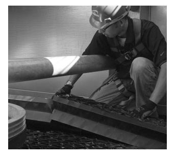
To remove the eliminator, stand inside the access panel and lift with two hands on an eliminator section, this will indicate where one section stops and another starts. Lift the eliminators at that intersection, removing two packs at one time (see image). Once the first two packs are removed, the remaining
