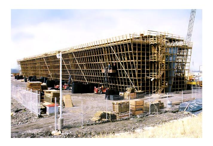
The diagonals brace the structure and carry loads to heavy-duty, hot dip galvanized anchor castings. The anchor castings transmit wind and/or earthquake loads from the structure directly into the foundation.
