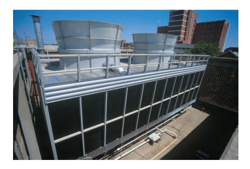
The Sigma F series crossflow cooling tower utilizes advanced composites and stainless steel for excellent durability and corrosion resistance in a truly cost-effective design.
