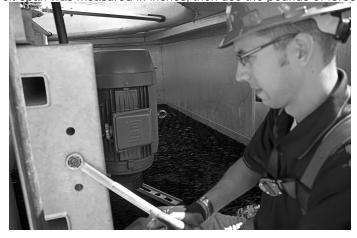
If the belt span was measured in centimeters, then use the kilograms of force values. If specific tensioning instructions are provided with your tensioning tool, those instructions should be used instead.
